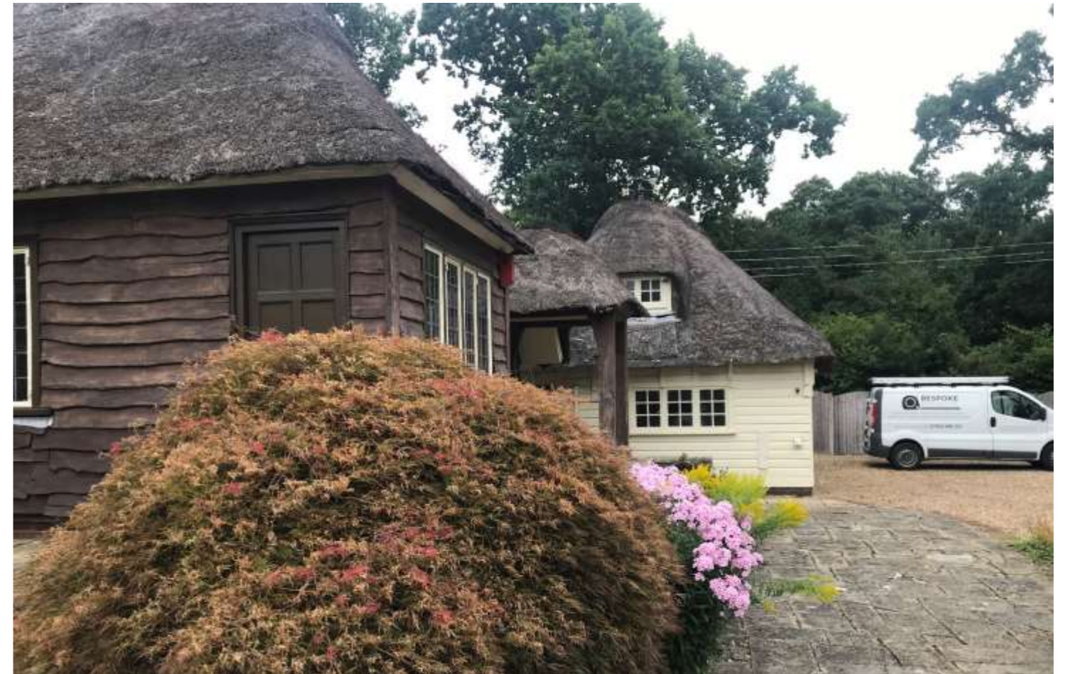
Photo 13: The view towards the front entrance from the garden, looking east.
