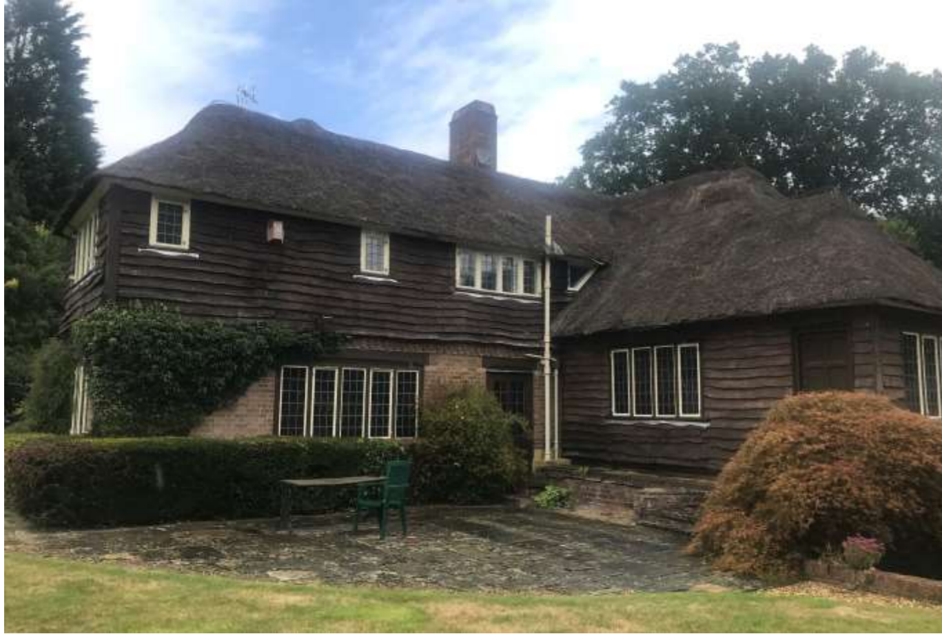
Photo 3: View of Arrow Cottage from south
