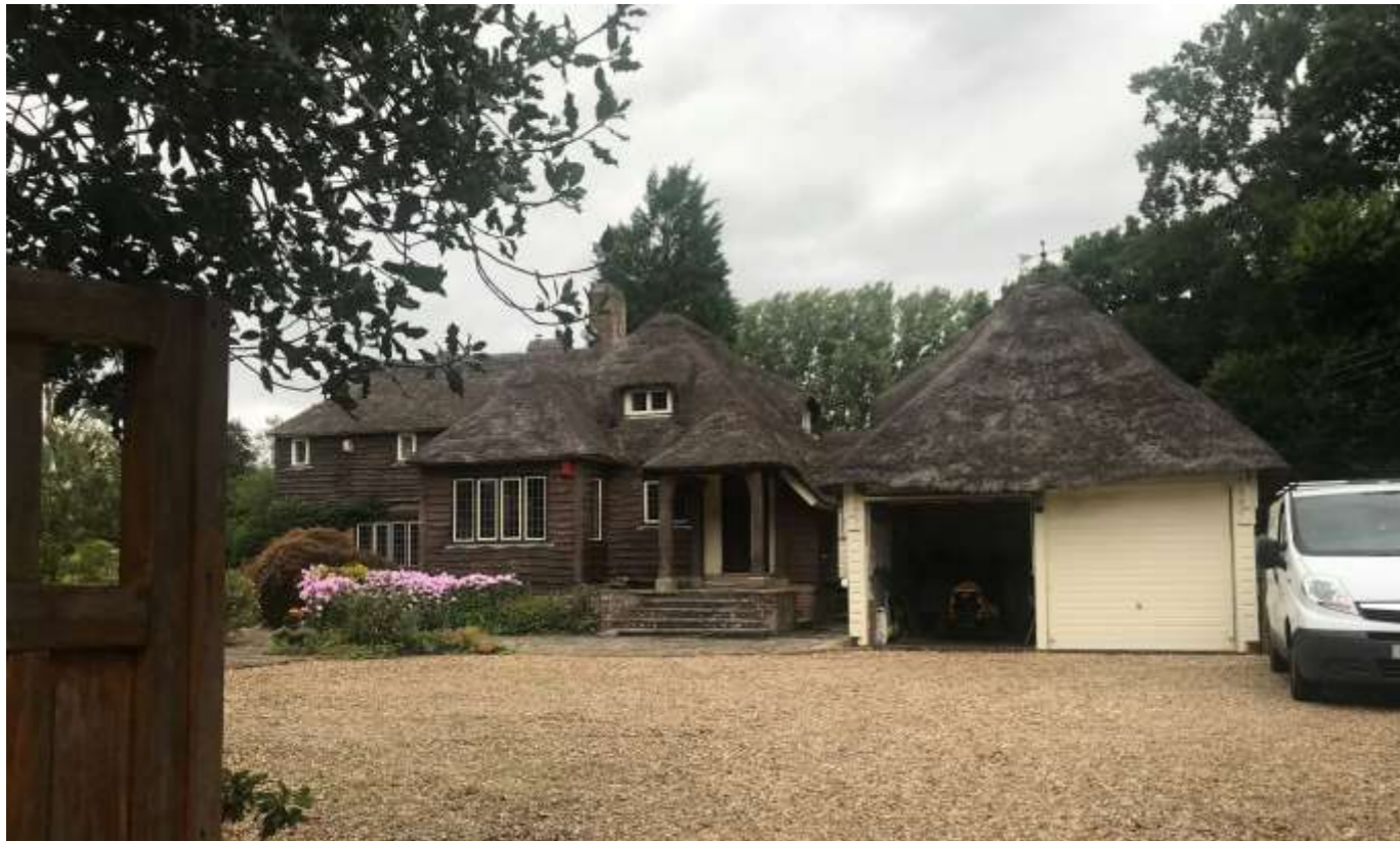
Photo 5: View of Arrow Cottage from south east (the main gated entrance)
